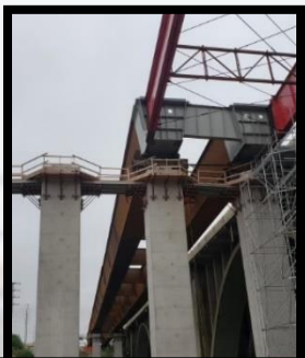
Credit River Bridge
